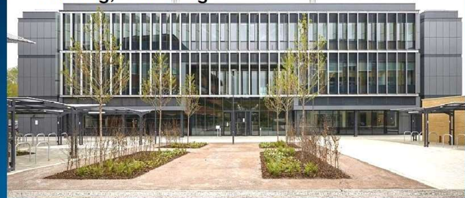
National Research Facility for Infrastructure Sensing, Cambridge
