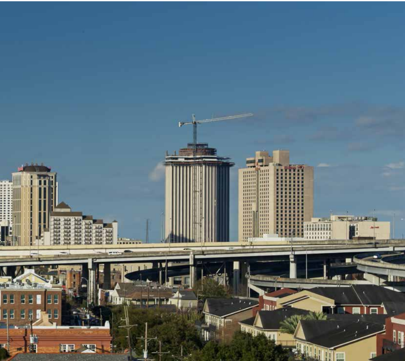
Elevated freeway through New Orleans
